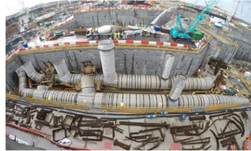
Conventional Island Unit 1 – CRF Inlet Trench
