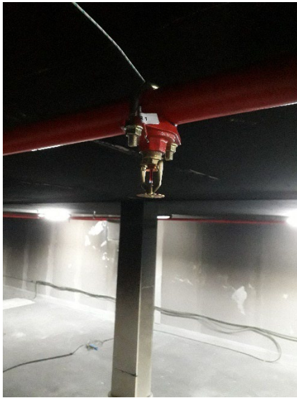
Detail residential sprinkler head
