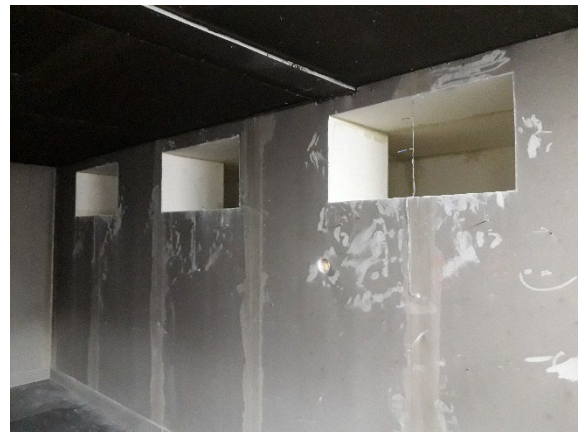
Exhaust openings in the common area
