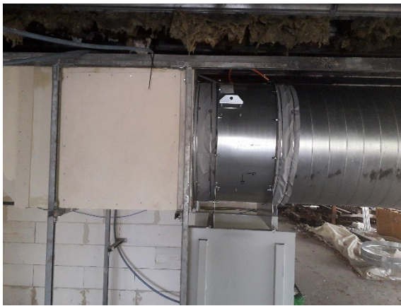
Detail rectangular duct – fan – circular duct
