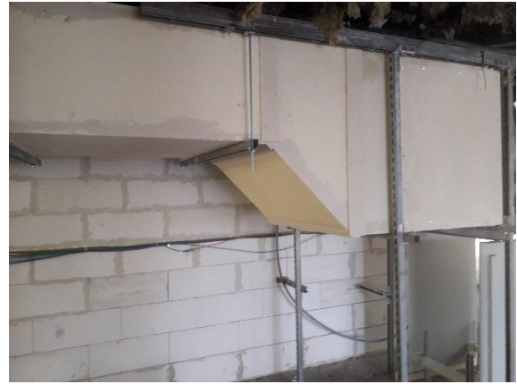
Transition rectangular duct to fan
